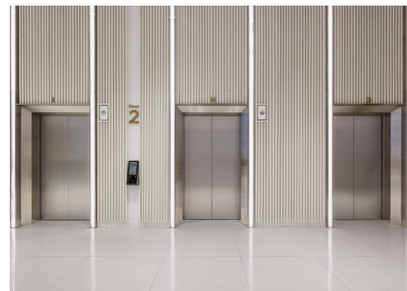
Elevator, Fig. S4
